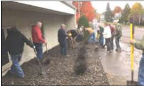
A group of 12 got together on the cold, drizzly morning of October 6 to dig up the stone along the side of the building, lay plastic sheeting and a protective layer and re-spread the stone to help correct the lower level leaks.
