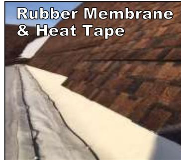
**GOOD NEWS:** Kulp's of Stratford finally arrived Tuesday, Dec 4 to fix the leak above the cry room and back coat rack where the steep Worship Area roof meets the flat Fellowship Area roof. They removed three feet of shingles, 'welded' four feet of membrane to the existing flat roof membrane and attached new shingles — as proposed.
