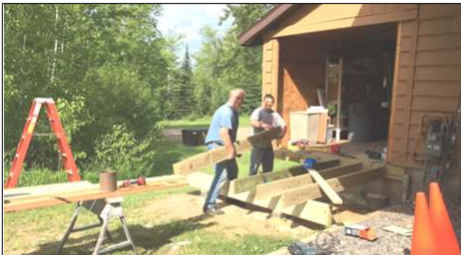
Trinity Lutheran members install a new Kitchen door and loading dock at Fortune Lake Lutheran Camp. Below: The old kitchen door and the new one with a loading dock and ramp!
