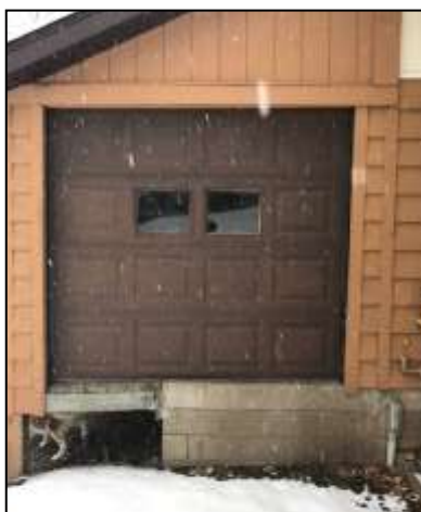
A new Double Door and Loading dock for the kitchen will be put in by Trinity Lutheran volunteers the weekend of June 9-10.
