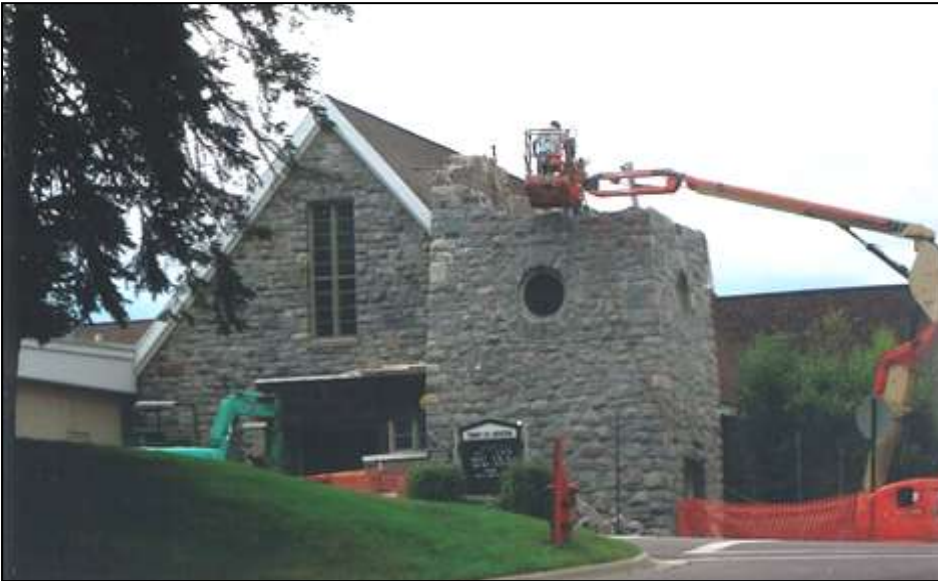
Above: Removal of the Bell Tower in 2013. Below: Trinity's Production of "To the Castle"
